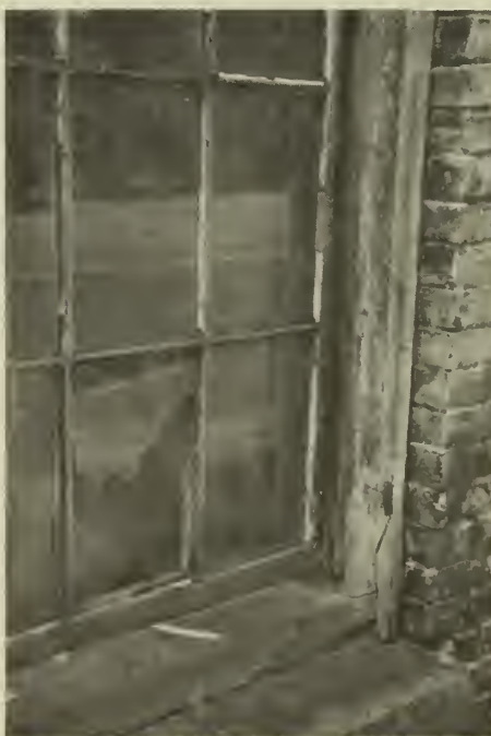
Figure 7. The retention of the exposed outer face of the historic wooden frame and the sill detailing were important qualities of the window treatment. Before and after photos: Charles Parrott
